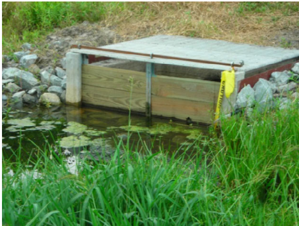
Figure C-6. Outlet varied with weir boards.
