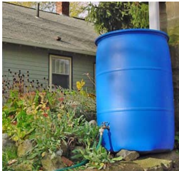
Source: Massachusetts Stormwater Handbook Figure 5-8. A 55-gallon rain barrel collecting rainwater from a residential rooftop.
