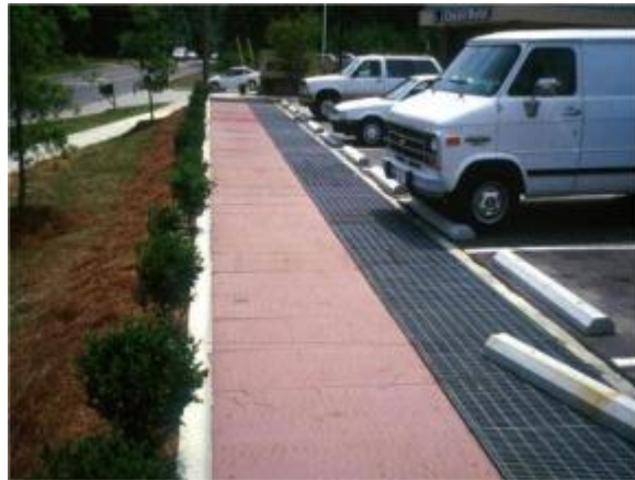
Figure 5-5. Below ground Delaware style sand filter installed in a parking lot.
