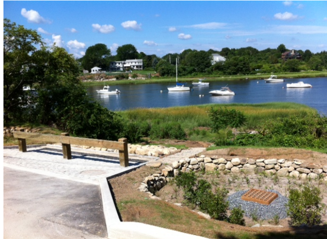
Source: Maureen Thomas, Town of Kingston Figure 1-2. Rain garden off of Delano Ave. in Kingston, MA.
