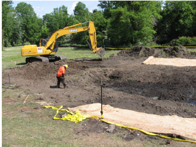
Figure 5-14. Heavy equipment (especially wheeled equipment) should be operated outside the excavated area to prevent compaction.
