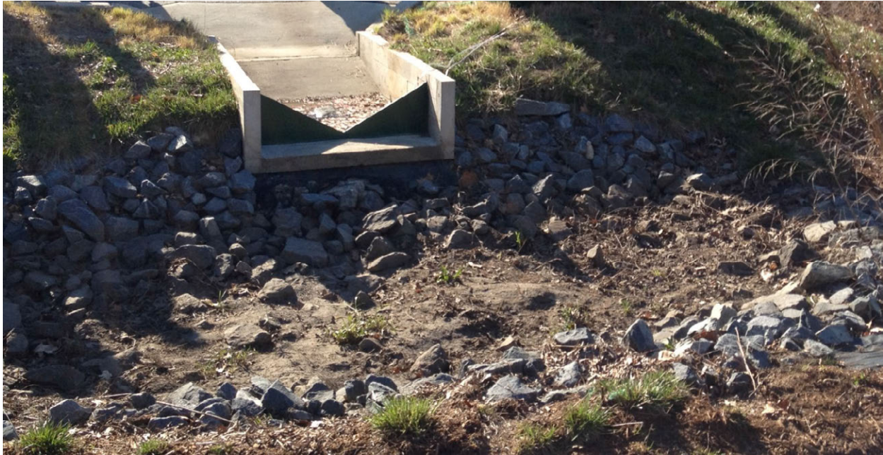
Figure C-10. Inlet curb cut with a v-notch weir.
