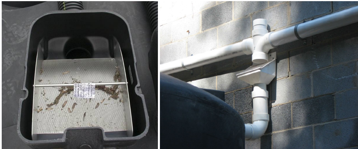
Figure C-5. Self-cleaning inlet filters.
