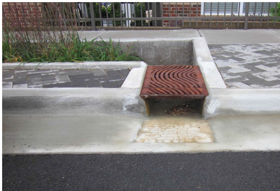
Figure C-2. Inlet sump to remove gross solids.
