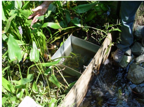
Figure C-7. Outlet with a trash rack.
