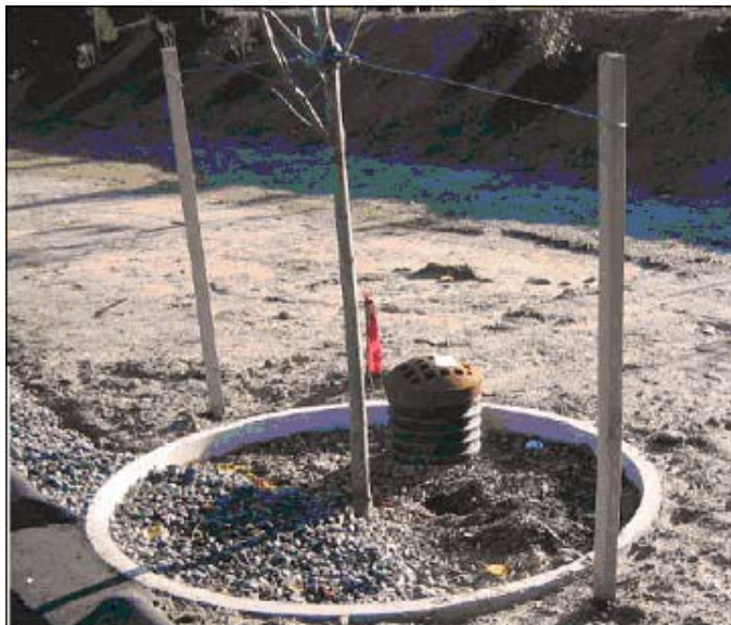
Figure 5-4. Newly constructed tree box filter.
