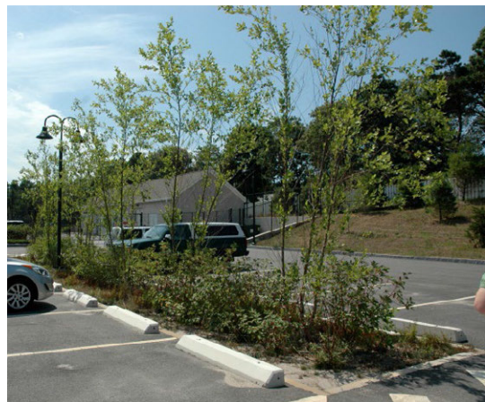
Figure 4-1. Bioretention cell (Cape Cod).
