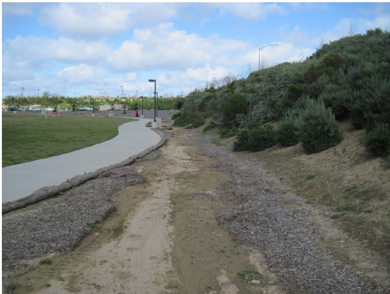
Figure C-3. Erosion caused by excessive flows in a bioswale.
