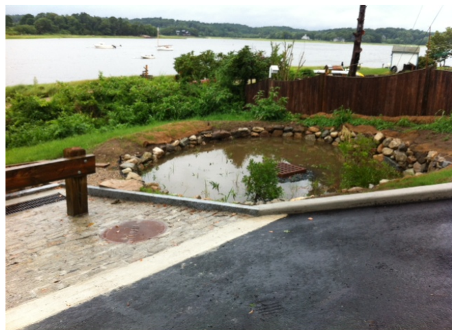
Source: Maureen Thomas, Town of Kingston Figure 1-3. Rain garden off of Delano Ave. in Kingston, MA during a storm event.
