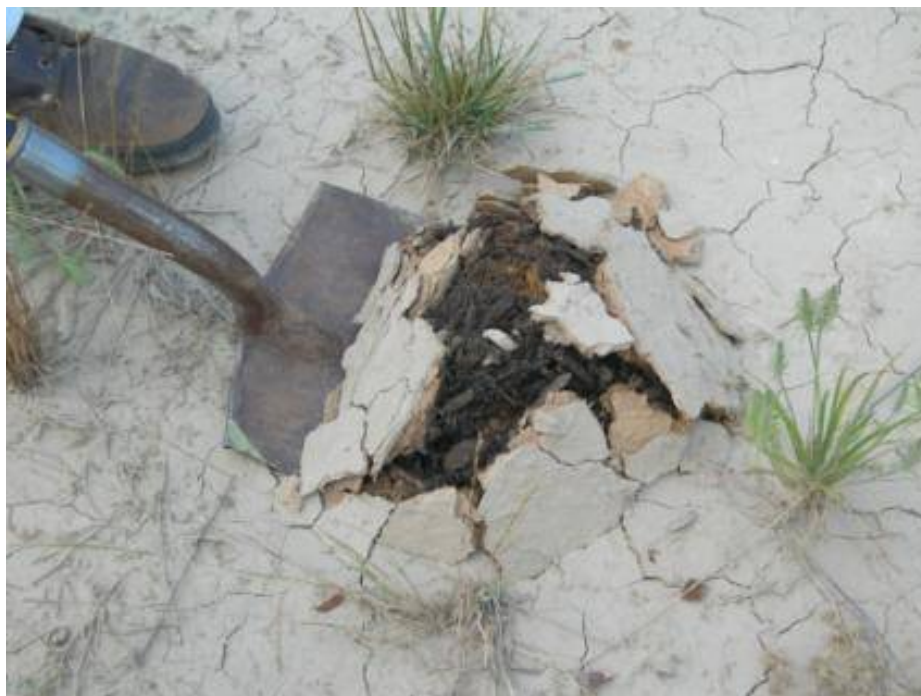
Figure C-1. Bioretention area clogged with sediment.
