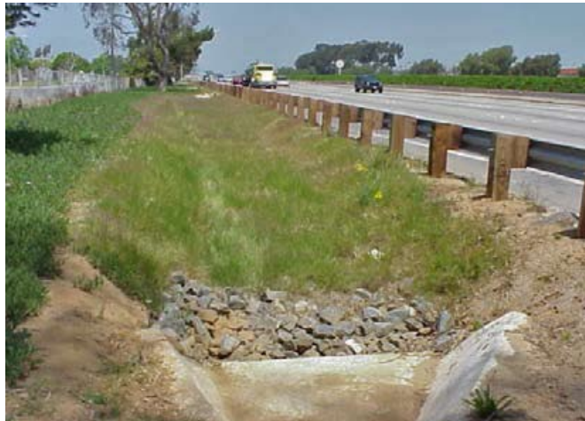
Source: Massachusetts Stormwater Handbook Figure 5-6. Grassed swale adjacent to a highway.
