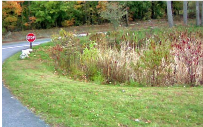
Figure 5-3. Constructed stormwater wetland with wetland vegetation.
