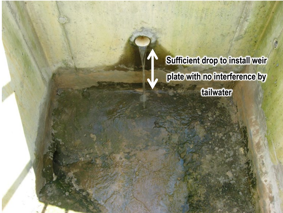
Figure C-13. Example of a bioretention underdrain outlet with sufficient drop to install a flow monitoring weir without encountering tailwater.
