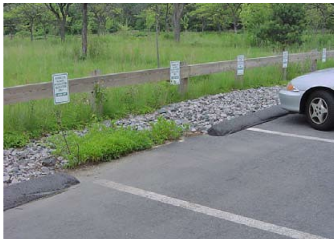
Source: Massachusetts Stormwater Handbook Figure 5-1. Vegetated filter strip at the edge of a parking lot.
