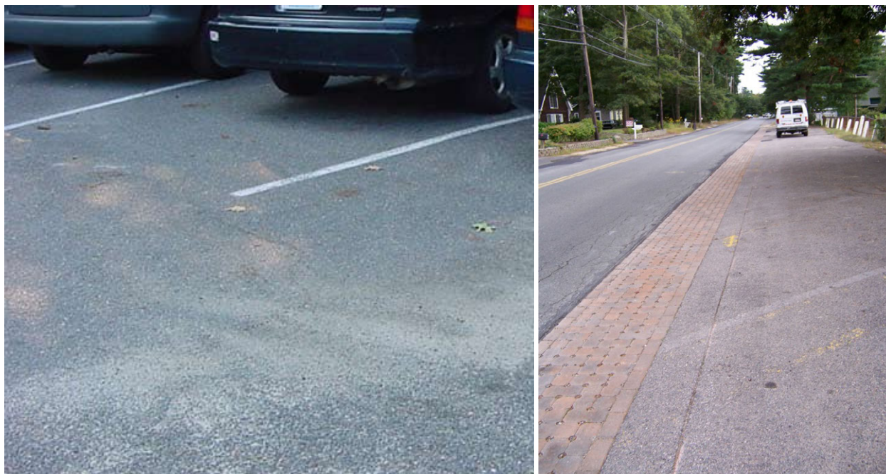
Figure 5-10. Porous asphalt parking lot and permeable interlocking concrete pavers in the right-of-way.
