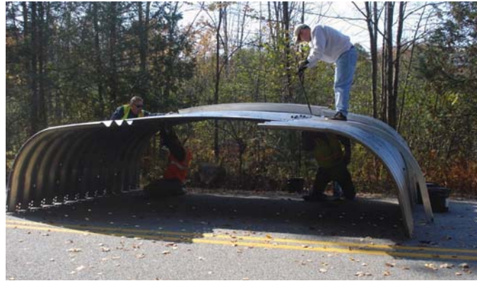
Figure 3-2. Gray Public Works and CCSWCD staff builds the bottomless arc culvert on site.
