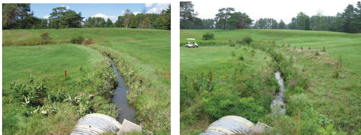
Figure 5-3. Riverside Golf Course 17th hole stream corridor BMP: before (L), after (R).
