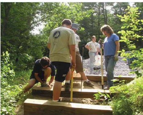
PRYCC crew members install infiltration steps on an eroding swimming hole access trail adjacent to a local road.
