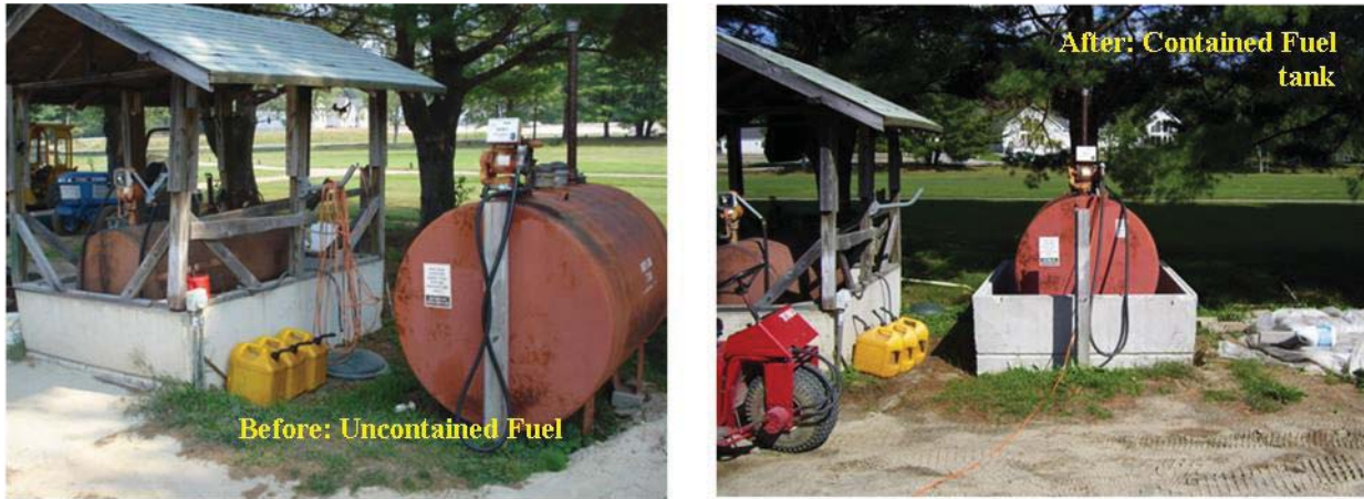
Figure 5-4. River Meadow Golf Course fuel tank containment BMP installation (F. Bell).
