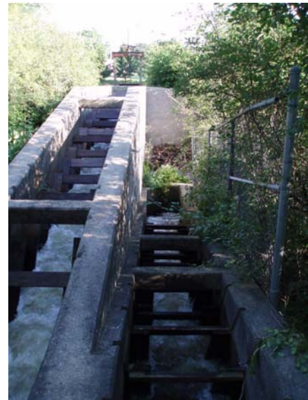
Photo 1-8. Denil fish pass at East Elm Street
