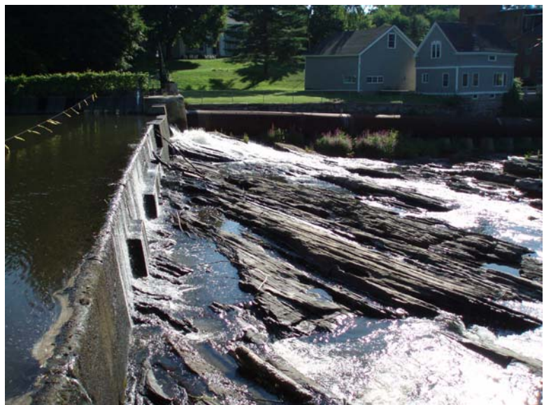
Photo 1-3. The Bridge Street dam was installed atop a series of stepped ledges, and serves as a complete barrier to fish passage.
