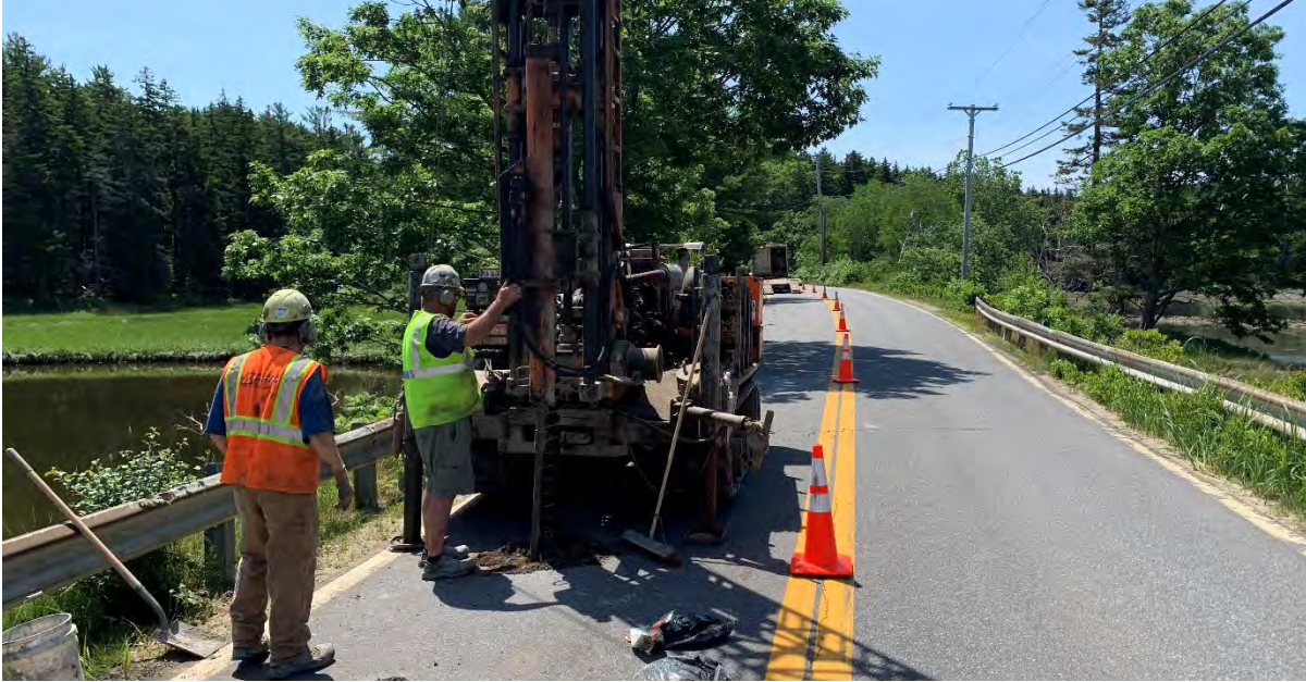
Boring/Probe Explorations being Performed on Small Point Road in July 2020
